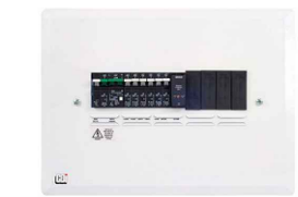
TYPICAL DISTRIBUTION BOARD
